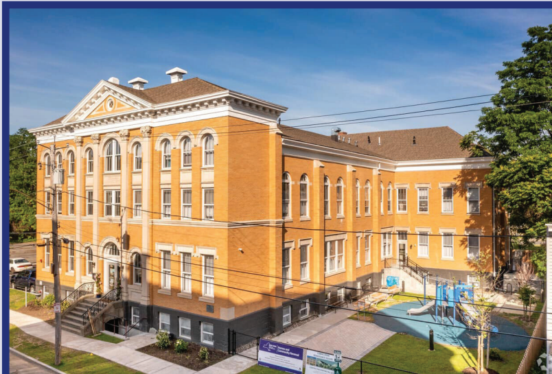
New $20 Million Senior Affordable Housing at Renaissance Square near Eastern Avenue.
